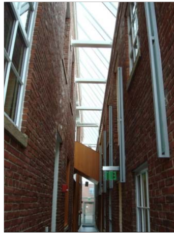
The unused expanse between buildings A and B was turned into a lightslot, reducing heat loss. (Harvard University Operations Services)
